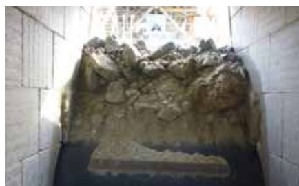
PRIMARY CRUSHED ORE 1500tph
